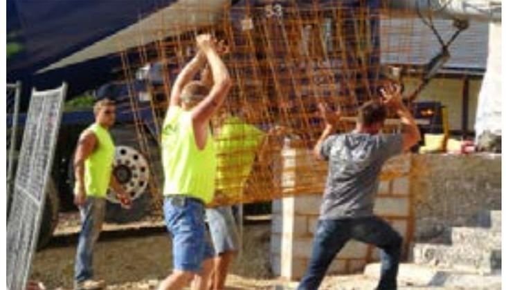
Above: Before the concrete truck arrived on August 18, workers mounted protective plastic on the front doors and carried reinforcing mesh to the top landing. Below: Maneuvering carefully, the truck poured concrete into a wheelbarrow, which was used to carry many loads to each section of the landing, covering the reinforcing mesh.
