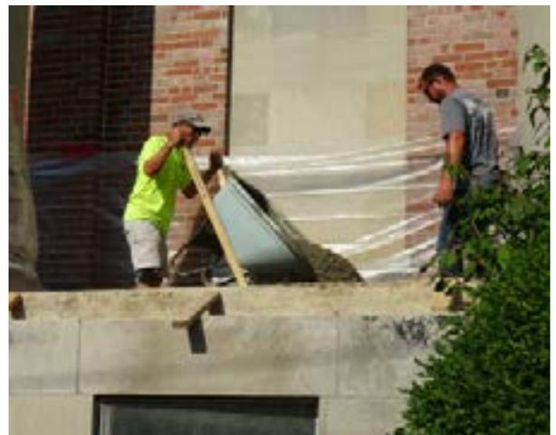
At right: On September 2, workers slathered the steps with steaming, tar-like rubberized asphalt, followed by protective mats meant to stave off water damage.
